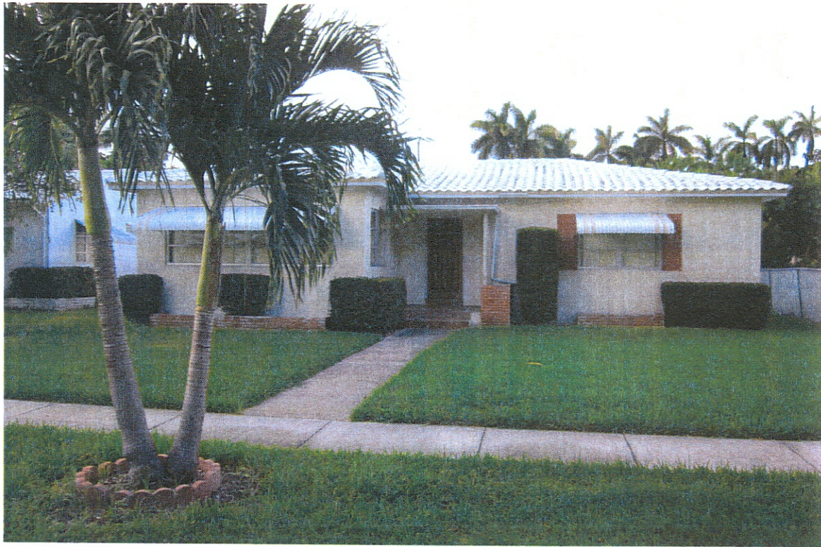
DIRECTLY WEST OF SITE
