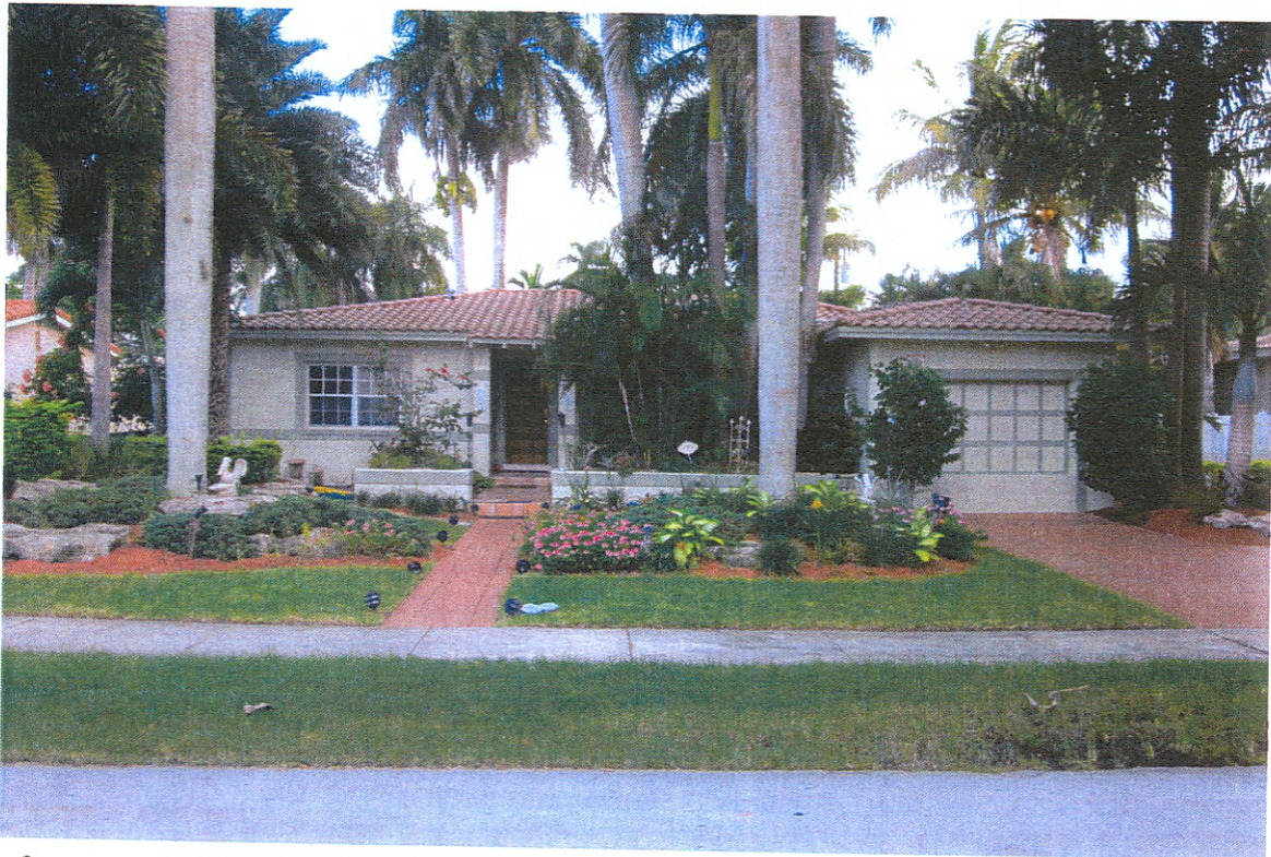
SOUTH EAST OF SITE
